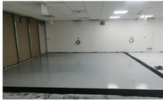
Anti Static Epoxy Flooring
