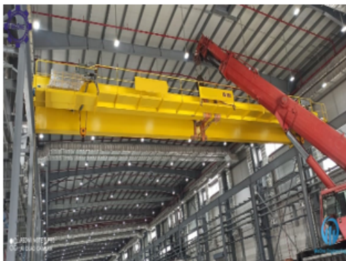
Installation & Commissioning of new Crane
